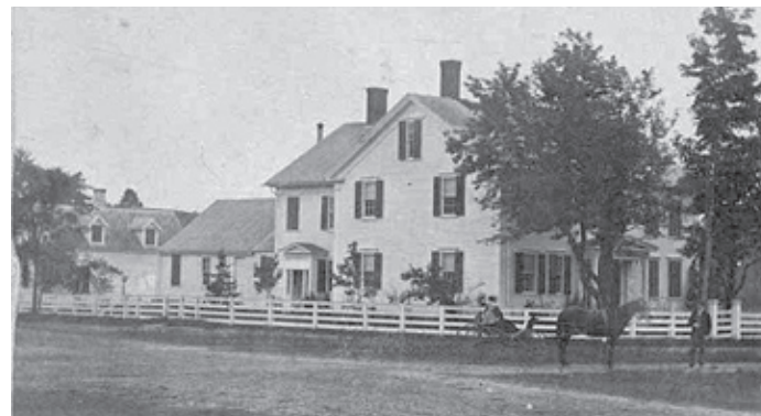
Joseph Cushing - Judge Edmund Parker House at 12 Main Street. Building on far left with dormers is Martha Moor House at 115 Boston Post Road. Historic image courtesy of Historical Society of Amherst, N.H.
