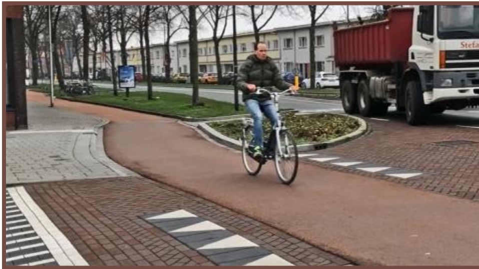
Figure 6 A sidepath/roadway intersection in which the sidepath's grade is maintained throughout (Wagenbuur 2011).
